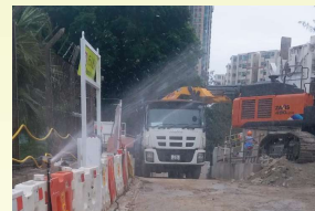
Spraying on haul road for dust suppression
