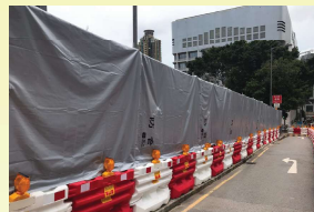
Erection of noise barriers
