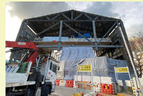
Construction of noise enclosure
